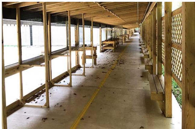
Continuous shooting line that shows the pistol bays after improvements
