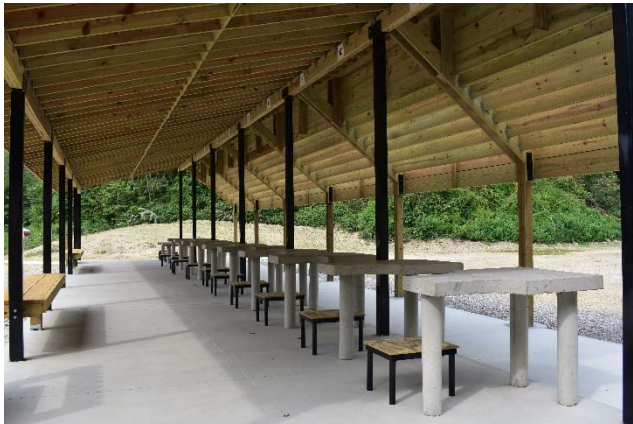
Newly constructed firing line and concrete benches at the rifle range
