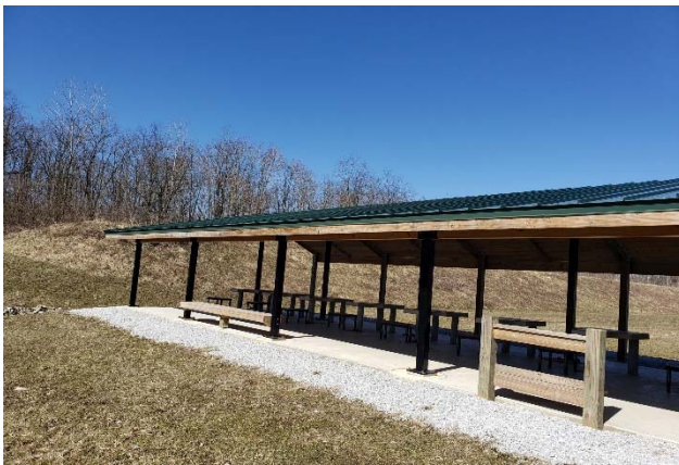
Newly constructed, covered shooting line with benches and gun racks
