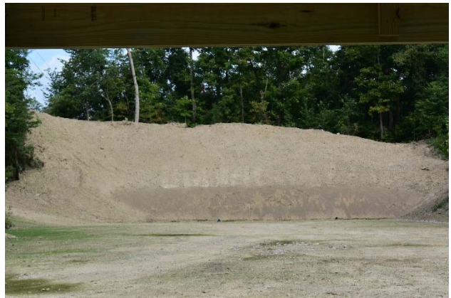
Reggraded and improved backstop at the rifle range
