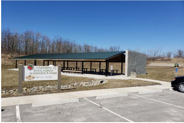
Shooting range parking lot and entrance after improvements made
