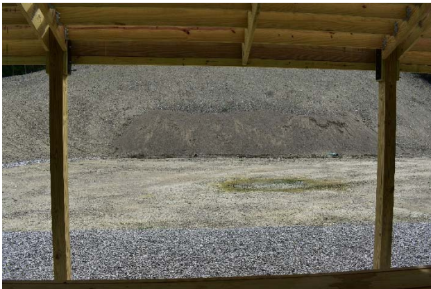
New backstop constructed at pistol range
