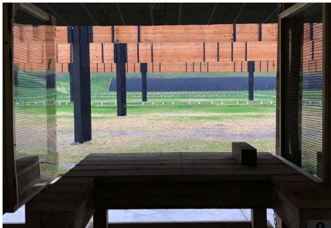
Looking down the 100-yard range with newly graded backstop and constructed baffles to eliminate "blue sky" for all shooters
