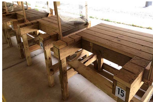
Newly constructed shooting benches at the 25-, 50-, and 100-yard ranges
