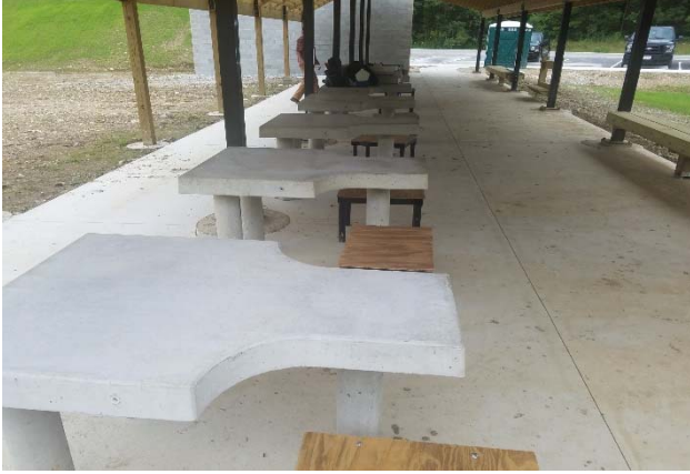
Newly constructed concrete shooting benches
