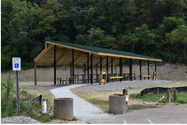
Newly constructed covered firing line at the rifle range
