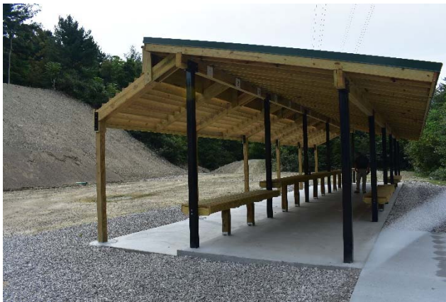
Newly constructed firing line at pistol range
