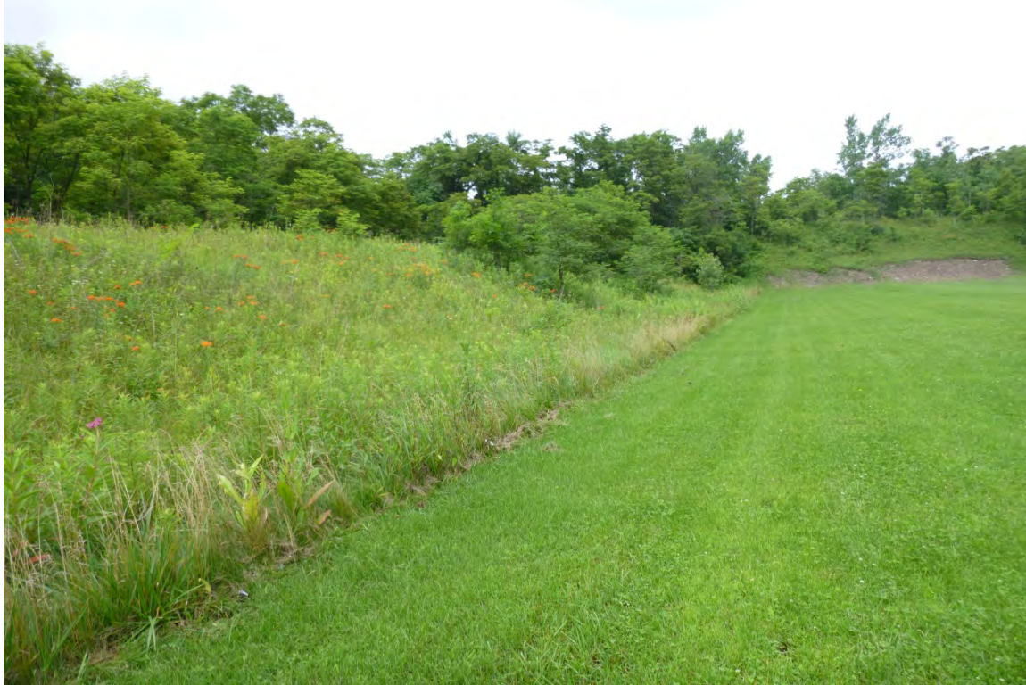
Photograph 3 Looking north at berm along west edge of range.
